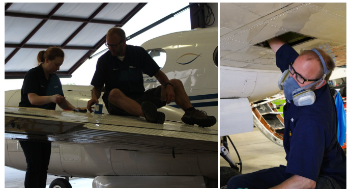
I worked with Mike and Jenny to install new fuel cells in this King Air 200 for Gospel Carrier International. One of the challenges of fuel cell installation is working in tight spots, sometimes with your fingertips at the limits of your reach.
